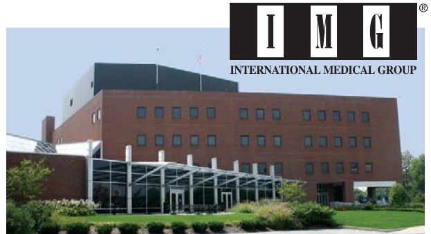
IMG World Headquarters, Indianapolis, Indiana
